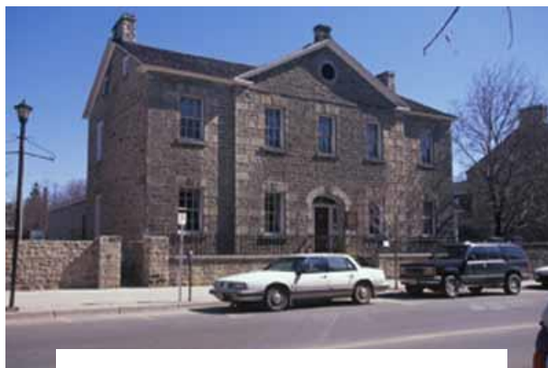
Matheson House National Historic Site
